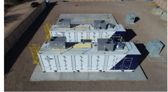
BESS at Punkin Center
