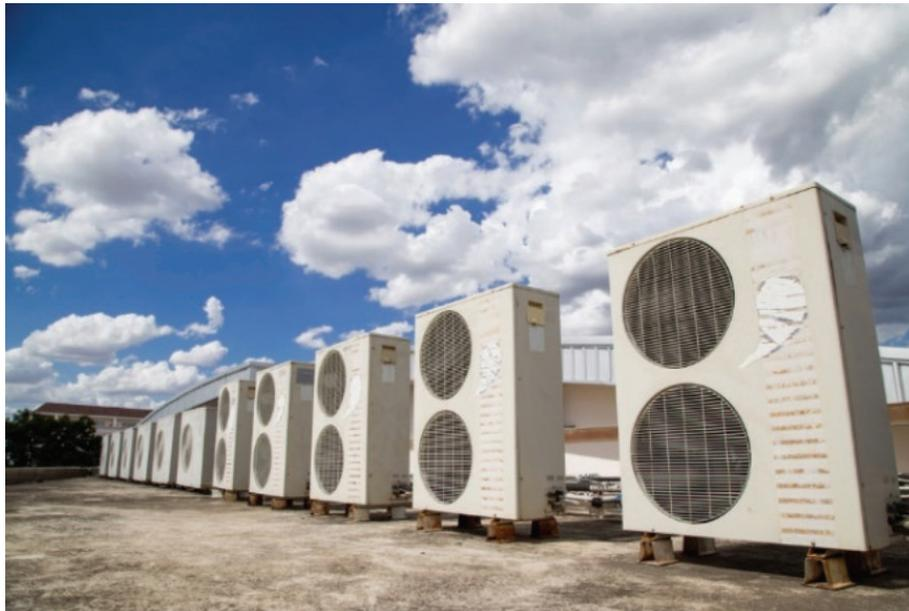
Figure 6 HVAC Rooftop Units. *Image courtesy CanStockPhoto.com.*
